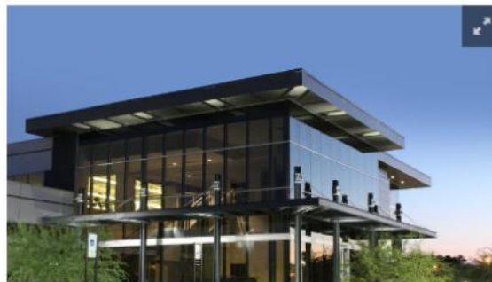
ViaWest's Nexus building in Tempe.
